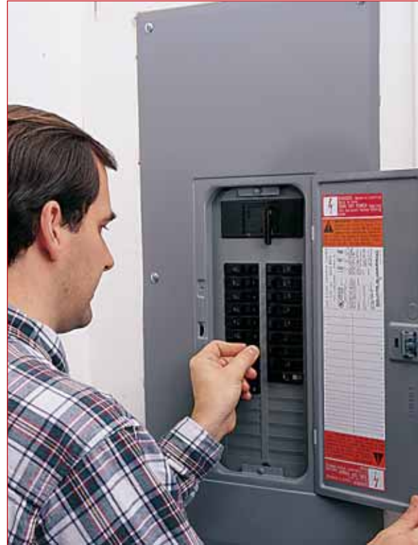
Load centers protect homes from electrical overloads and short circuits. Photo courtesy Schneider Electric/Square D
