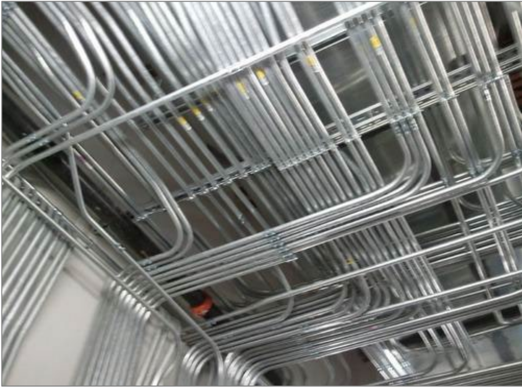
.conventional pipe & wire..
